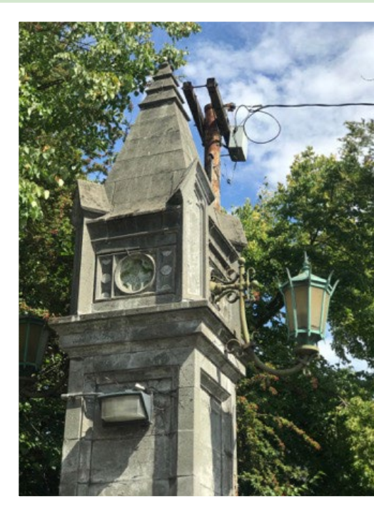
Restored Lantern on the Montlake Bridge
