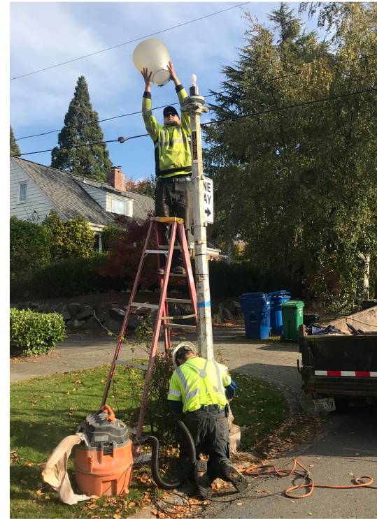
Contractors removing the historic lamp posts, Fall 2019.
