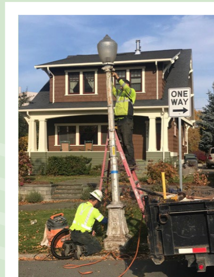
Removing one of the lamp posts.
