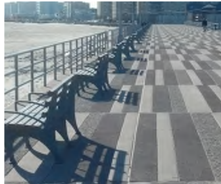
Concrete Paving with Special Finish
