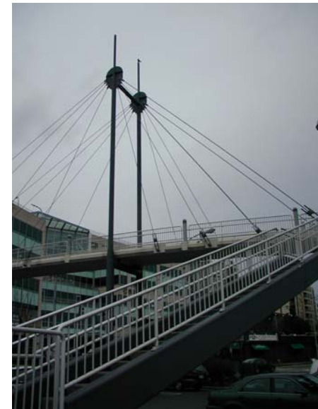
Galer Street Pedestrian Bridge
