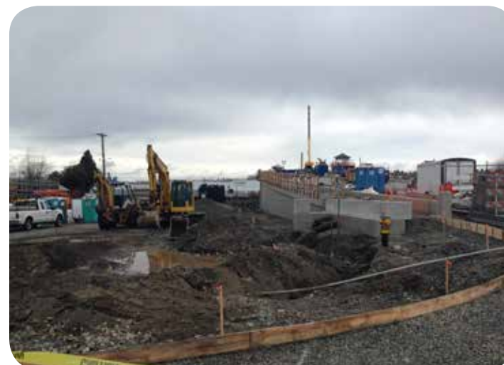
Parts of the site being prepared for bridge material staging
