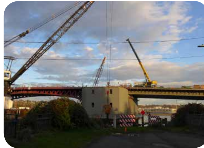
The site looks out over the new South Park Bridge
