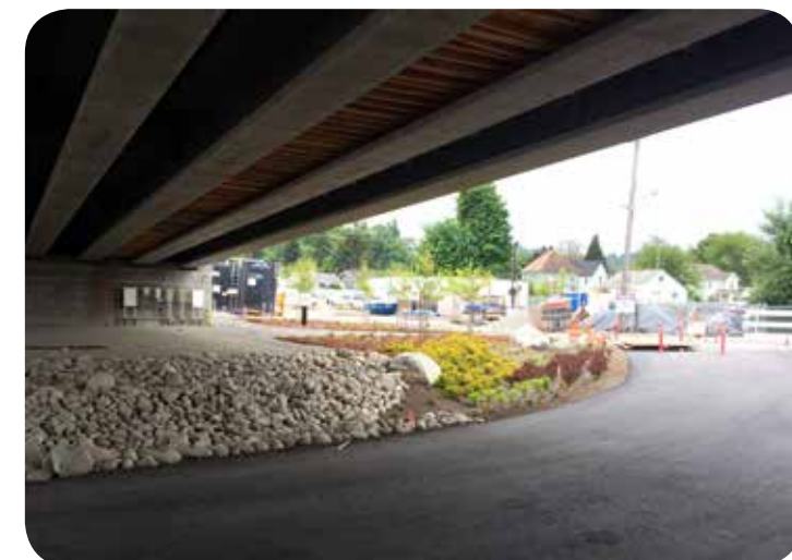
Look out at the north end of the site from under the bridge
