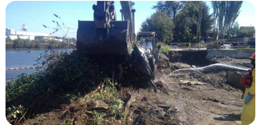
Beginning of Site Clearing
