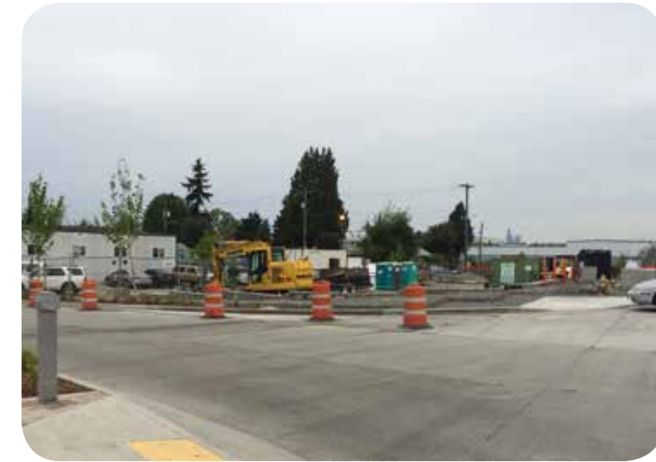
Looking north at the plaza, staging materials are laid out
