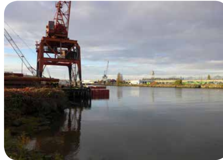
Looking north from the site out over the river
