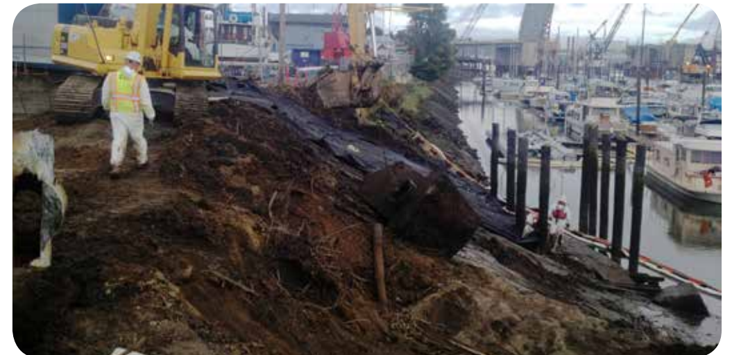
Removing of Contaminated Soil
