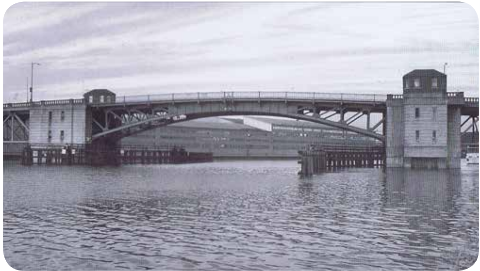
The previous South Park Bridge
